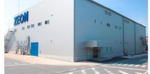
SGCNT mass production plant (Zeon Corporation Tokuyama Plant)
